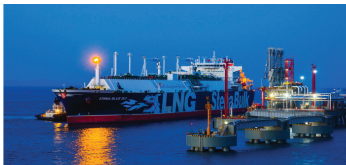
Zhoushan LNG terminal in the Zhejiang Free Trade Zone
