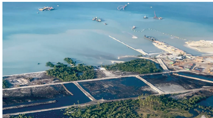
Plant site on Afungi Peninsula near the port of Pemba
