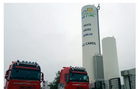
LNG vehicle fuelling station in Bakum, Germany.
