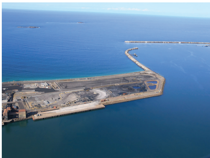
Work is to start on Port Kembla's receiving terminal. Photo credit...C Douch
