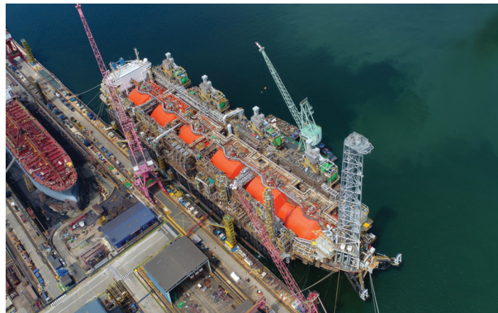
The 'Hilli Episeyo' conversion caused far less emissions than a newbuilding counterpart
