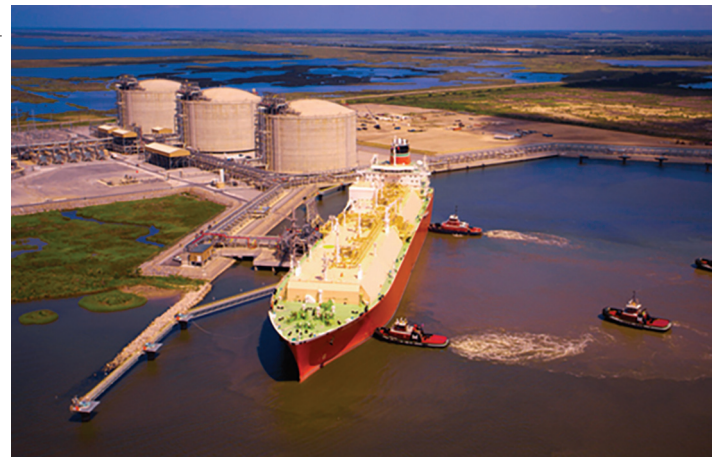
Cameron LNG is just one plant being inspected in the US Gulf in the aftermath of the hurricane
