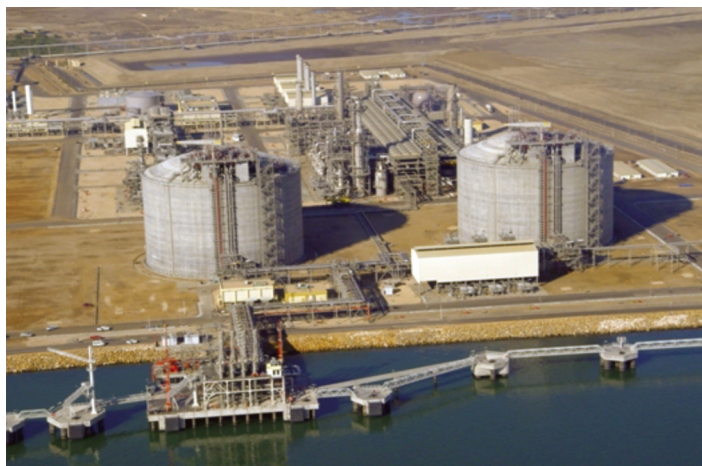
The compact liquefaction plant is east of Alexandria port
