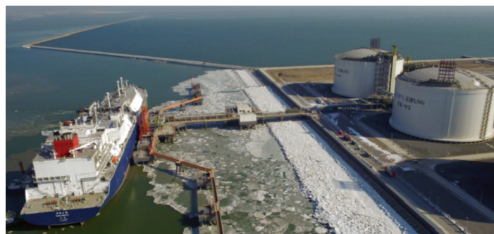
One of the company's regas facility in port of Tianjin
