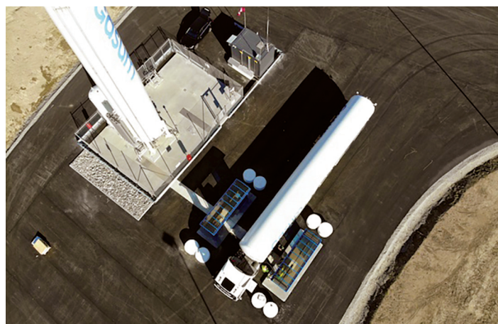
Birdseye view of Chart LNG compact station
