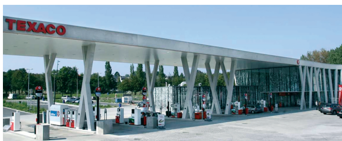
Liqual refuelling station
