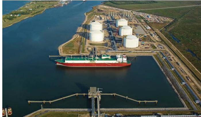
Calcasieu Pass LNG export project in Cameron Parish, Louisiana
