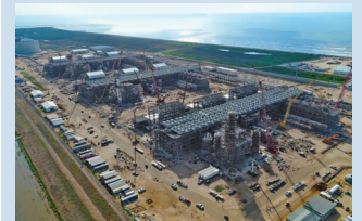
Freeport LNG during construction
