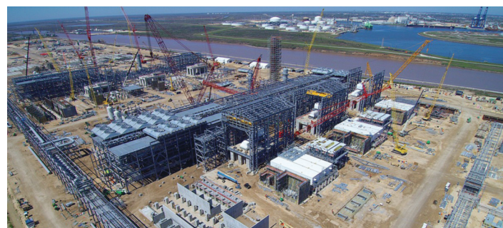
Construction of Freeport LNG Train1 at Quintana Island, Texas.
