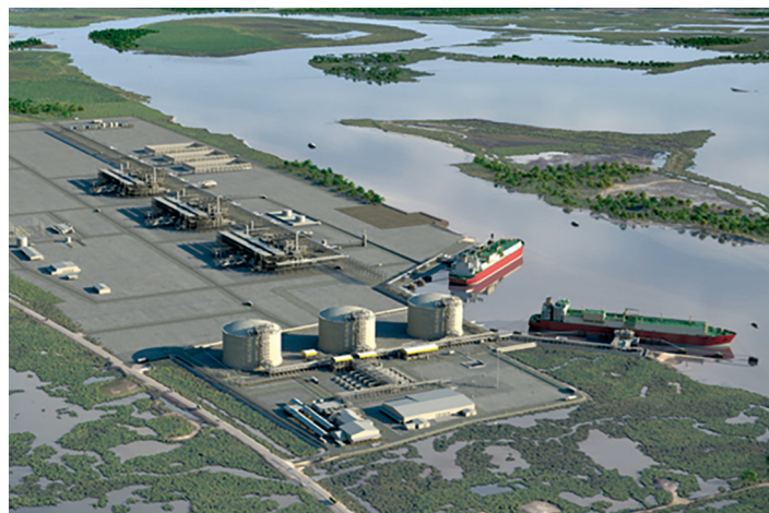
Mitsui joins Cameron Phase 2 development
