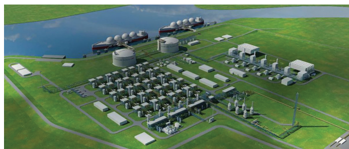
Venture Global's Calcasieu Pass project is now fully funded
