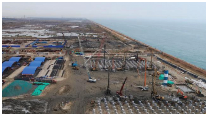
Tangshan-Caofeidian LNG facilities are being expanded
