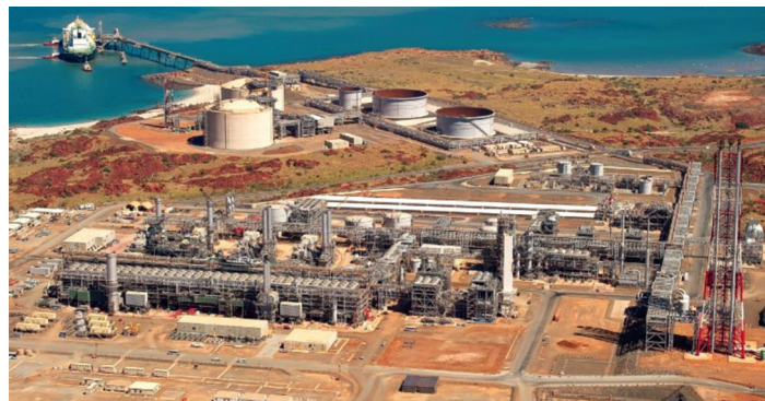
Normal service is resumed at Pluto LNG export plant
