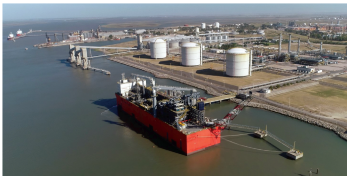
Production hull 'FLNG Tango' at Bahia Blanca in Argentina
