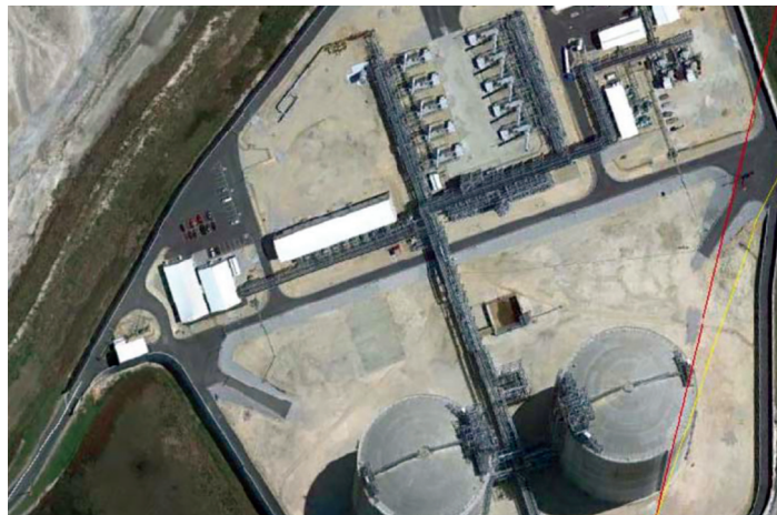
Aerial view of existing facilities at Pascagoula terminal
