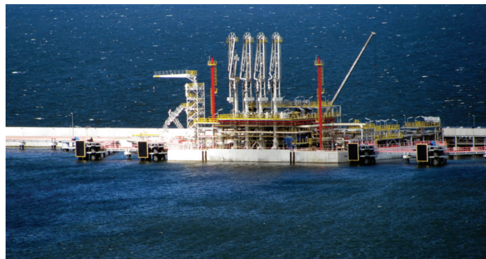
Polish regas facility at Swinoujscie on the Baltic coast
