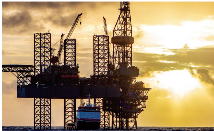
Platform and four wells located 60km offshore Trinidad
