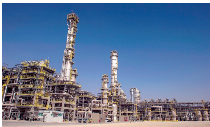
The 2.1-billion Saudi industrial gas complex built in Jazan
