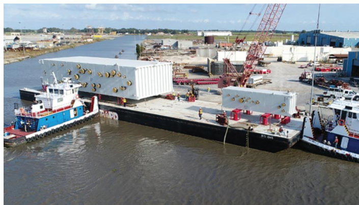
Chart's primary cold box fabrication location is a 40-acre coastal facility in Louisiana on Gulf Coast
