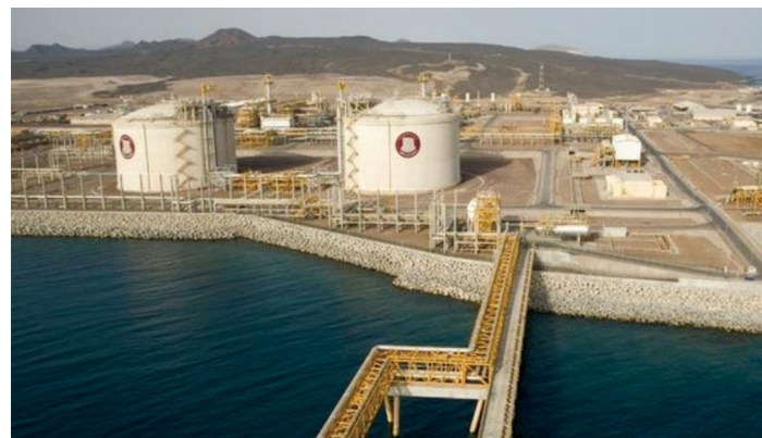
Plant is still intact after shutdown because of conflict
