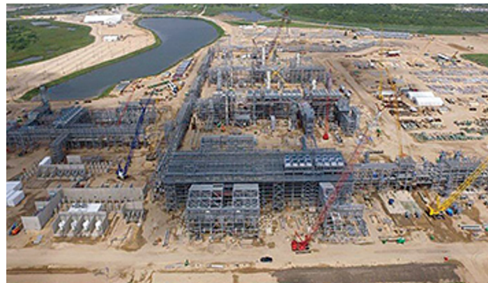
Chiyoda is also working on the Freeport LNG plant in Texas
