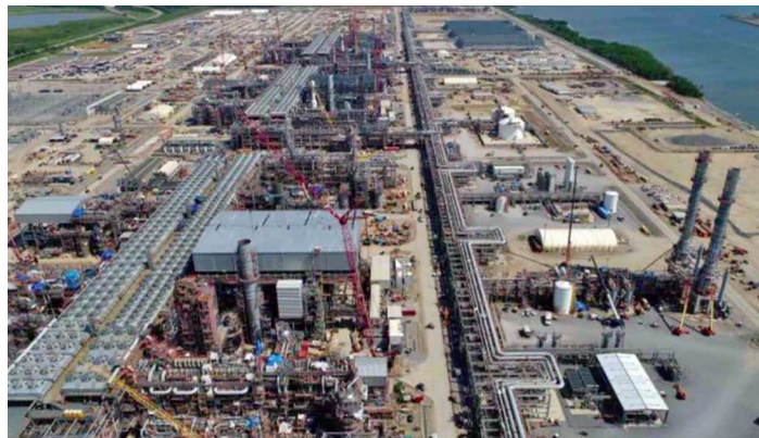
Sempra's Cameron export plant site in Louisiana
