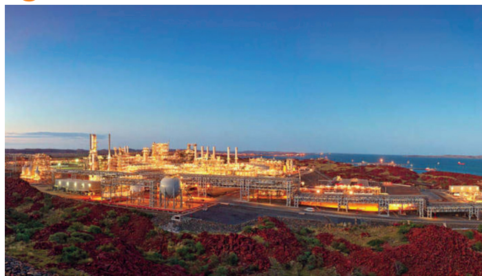
Scarborough gas field for Pluto LNG is next development
