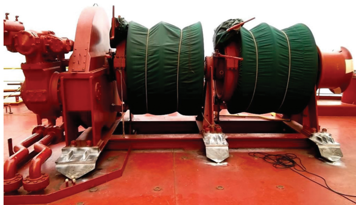
Harris Pye has completed mooring winch upgrades on two LNGCs
