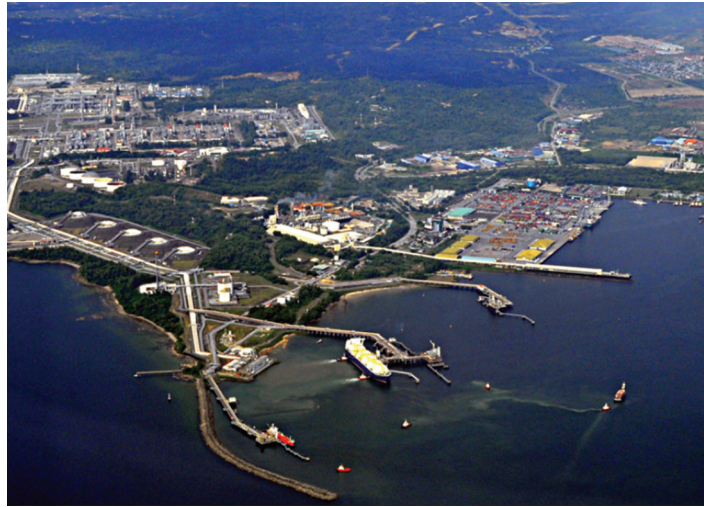
Bintulu Port and LNG plant in Sarawak welcome ships
