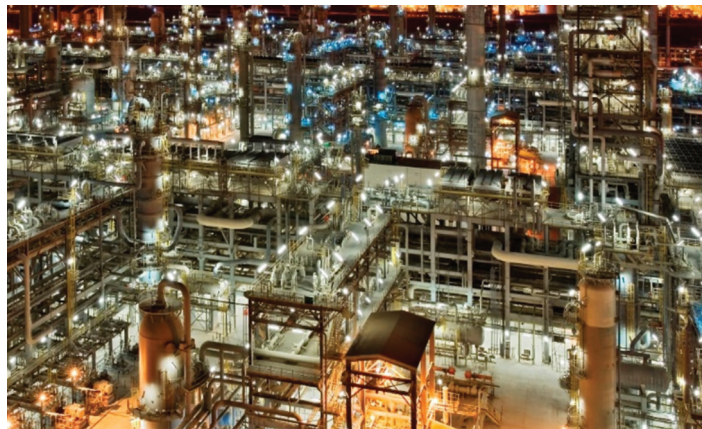
Qatar's Ras Laffan processing complex will be expanded
