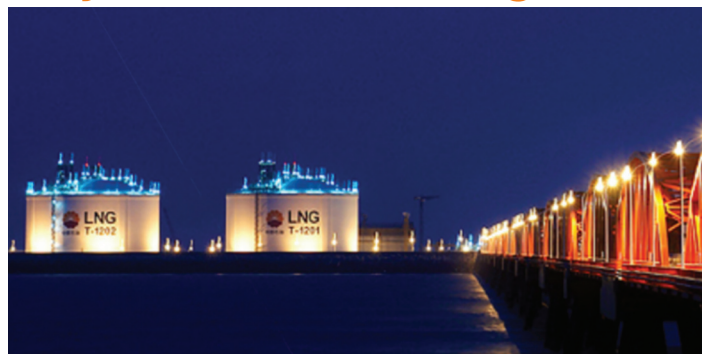
PetroChina import and regas facility at Tangshan
