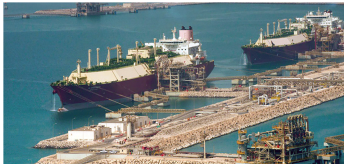
Carriers lifting cargoes at Ras Laffan complex in Qatar
