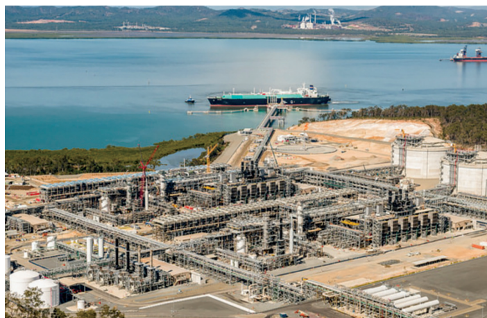
Santos-operated liquefaction plant on Curtis Island
