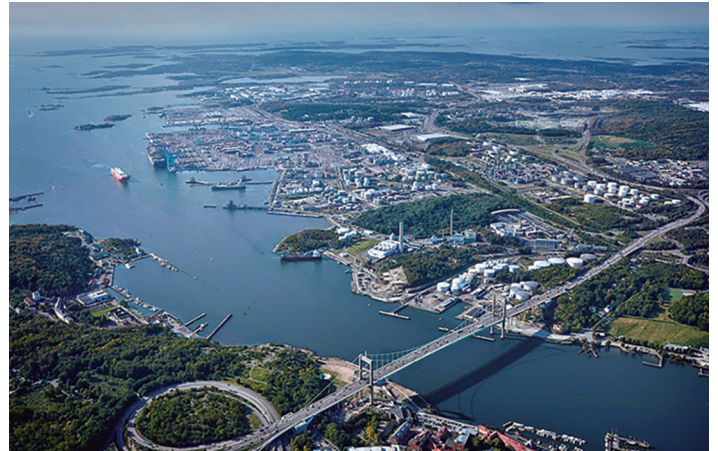
Port of Gothenburg
