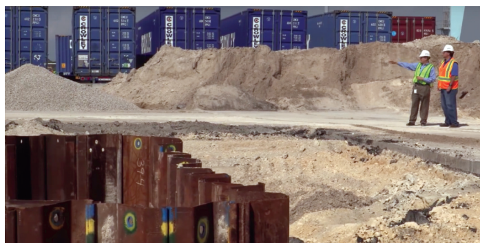
Construction is underway at the Jaxport site
