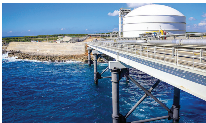
Terminal-1 within the AES Andres energy complex
