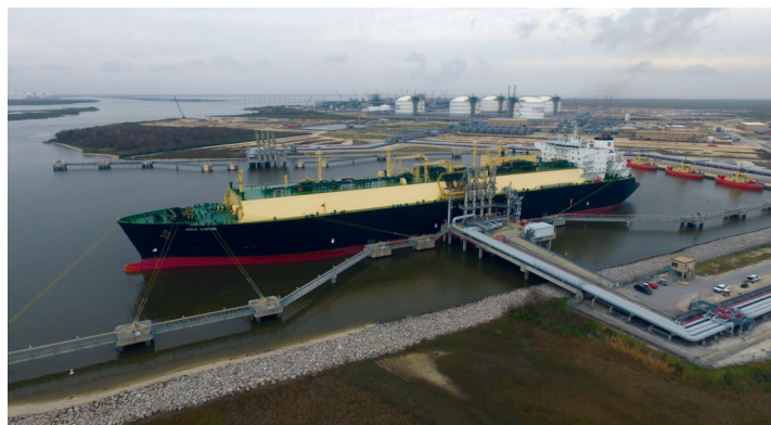
No damage was reported at Cheniere's Sabine Pass facility
