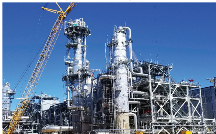
Liquefaction plant now in operation at the site in Maryland
