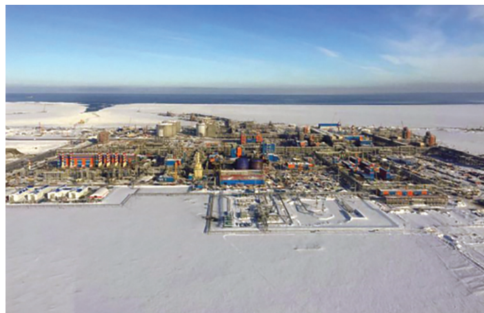
Liquefaction plant built in extreme conditions
