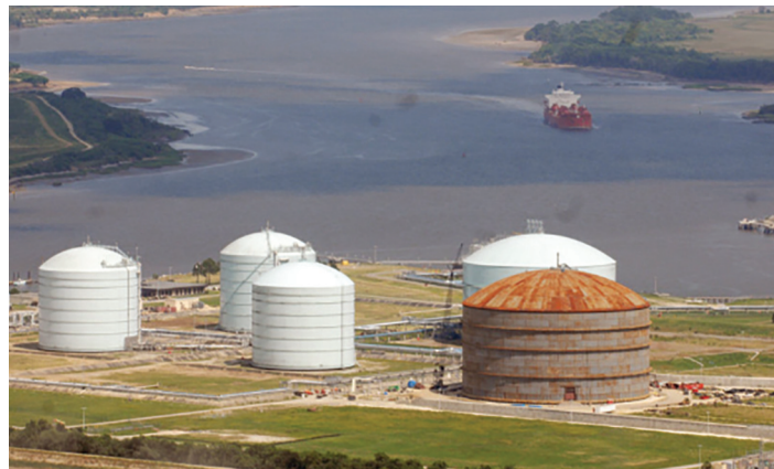
Existing terminal being turned into export plant
