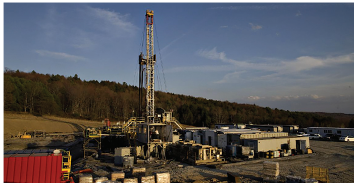
A drilling operation in Haynesville Shale in Louisiana
