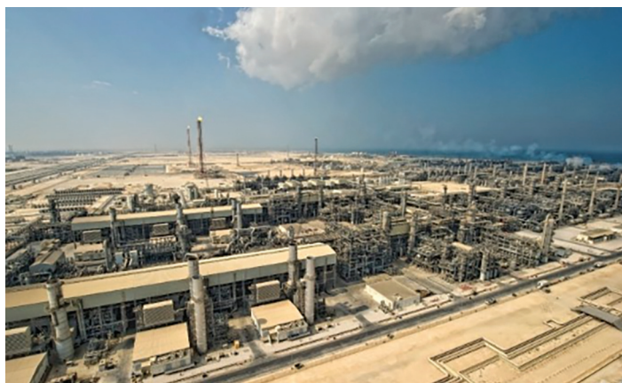
First Ras Laffan Train has been operating since 1997
