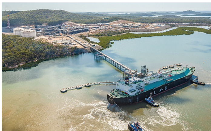
Gladstone LNG plant, one of three on Curtis Island
