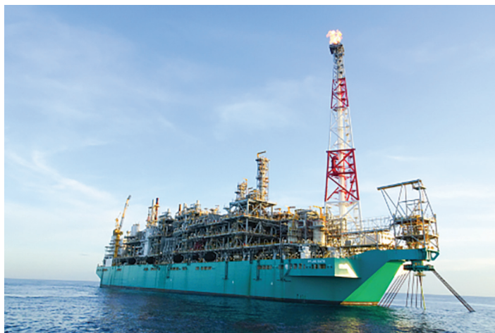
'PFLNG Satu' received feed-gas from Kanowit platform
