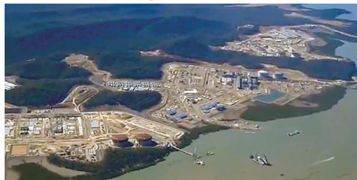
Aerial view of the three liquefaction plants on Curtis Island
