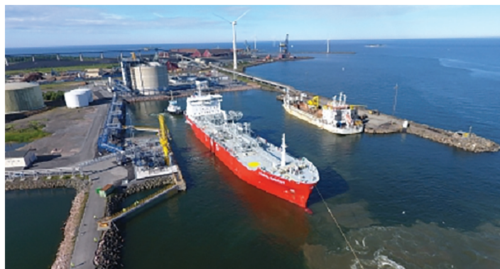
Newest European LNG terminal at Pori port in Finland
