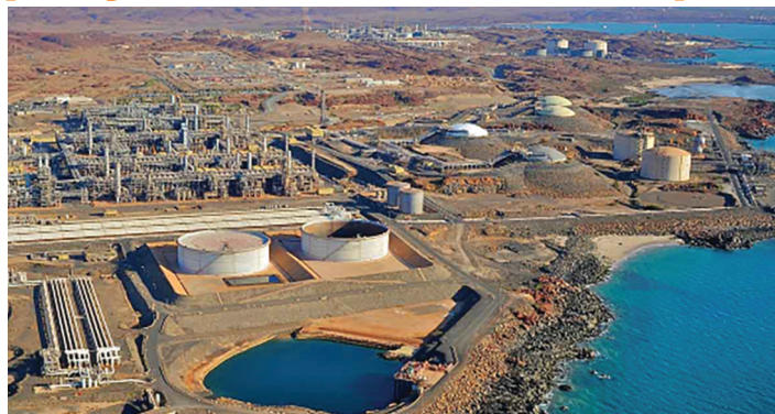
Woodside-operated Pluto liquefaction plant is located 190km northwest of the NWS export facility at Karratha
