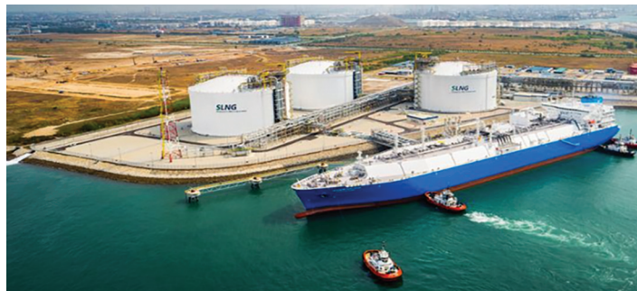
Jurong Island LNG terminal expansion is already envisaged
