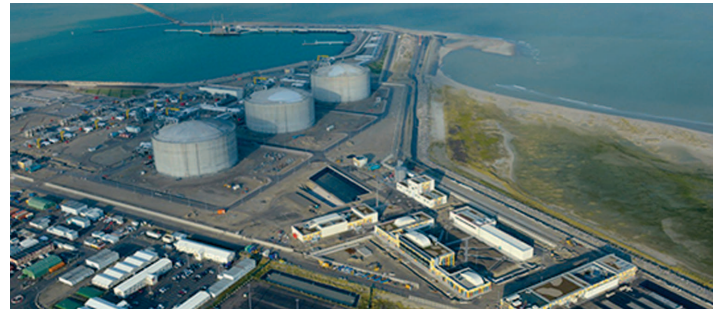
EdF will deliver cargo to new Channel terminal on July 8
