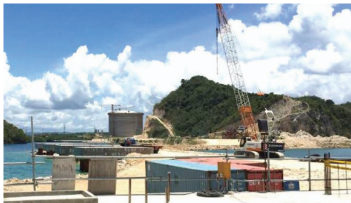
Pagbilao terminal will be able to handle 3 million tonnes
