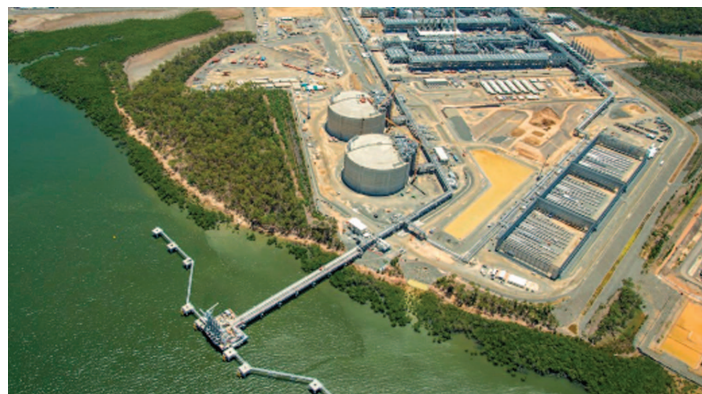
Australia Pacific LNG plant on Curtis Island in Queensland
