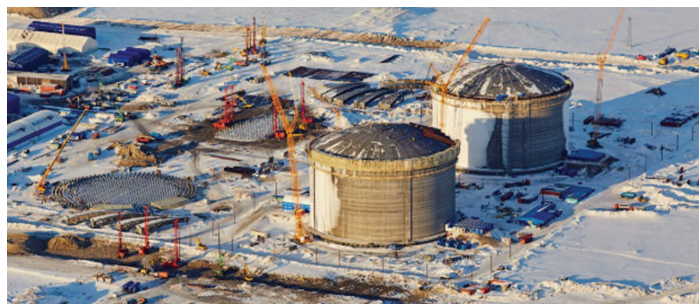
Plant under construction will have three Trains and storage
