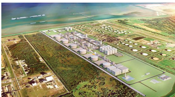
Render of Wilhelmshaven regas terminal
