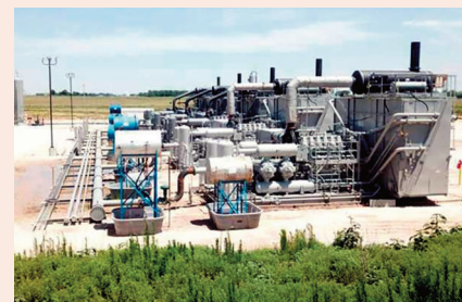
SGT-400 gas turbine core
