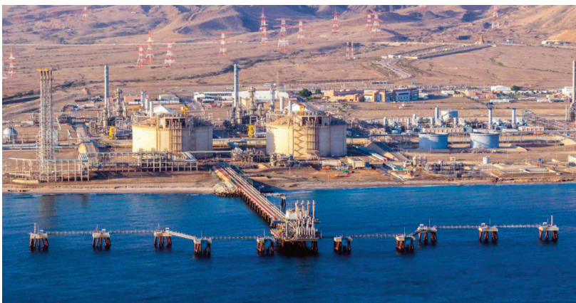
Oman LNG plans to add a third train at its Qalhat complex by 2029
