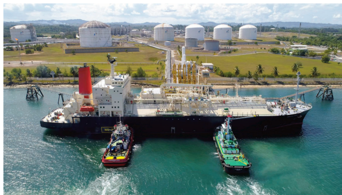
The 22.5 mtpa Bontang LNG terminal is one of the world's largest liquefaction plants
