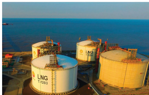
Chevron's Gorgon LNG trains in Australia
