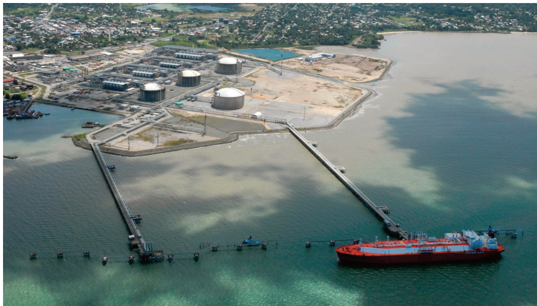
Tanker berths at Atlantic LNG's Point Fortin facility in Trinidad
