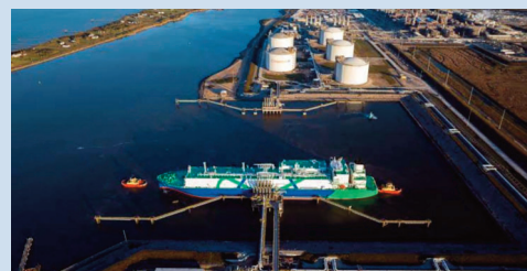
Carrier loading at Golden Pass LNG terminal
