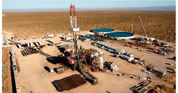
Fracking operations in the Vaca Muerta formation
