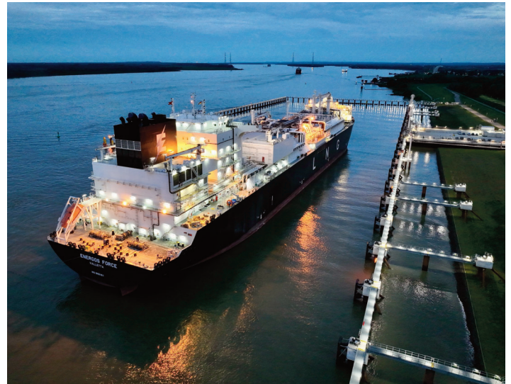
DET's Stade import terminal could help Europe's storage once commissioned
