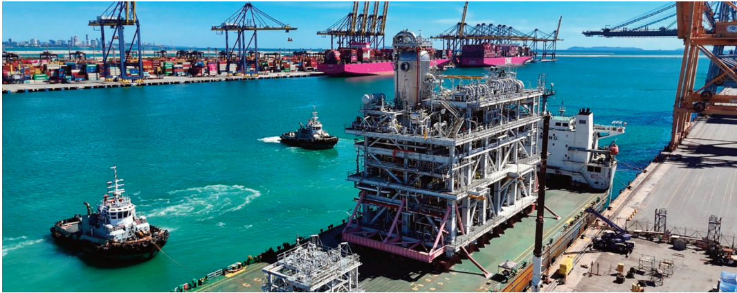
The last module for the Pluto LNG Train 1 upgrade has arrived on site
