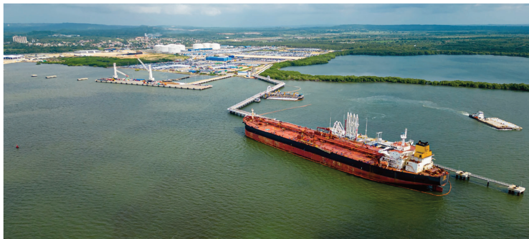
Puerto Bahía's new LNG terminal can be seen in the background
