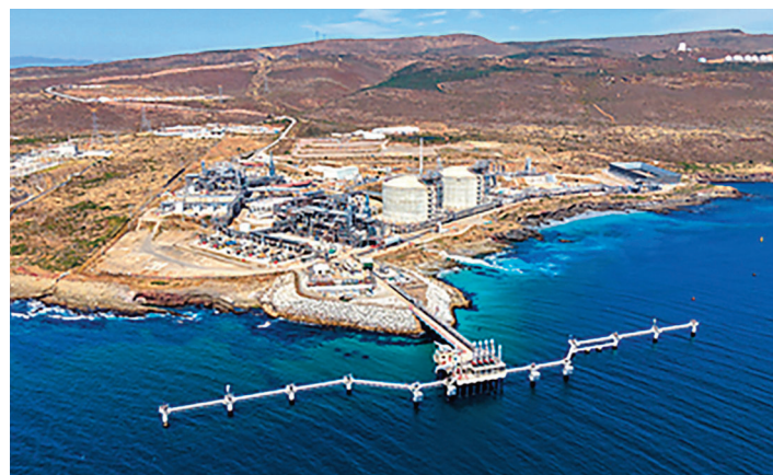
Sempra Infrastructure has announced ECA LNG production startup
