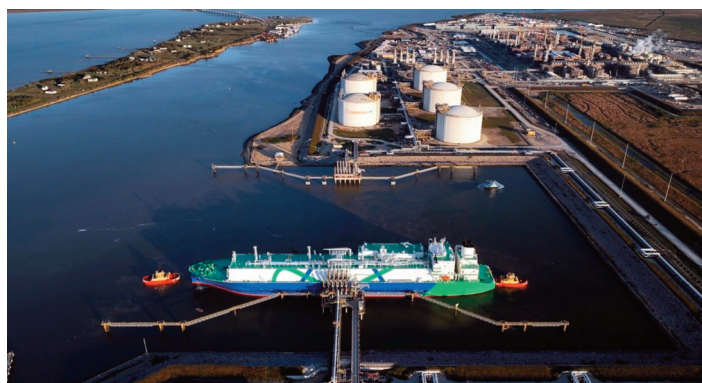
The commissioning cargo arrives at Golden Pass
