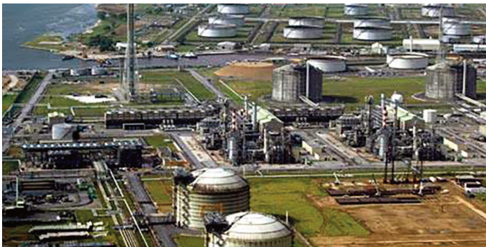
NLNG production complex on Bonny Island
